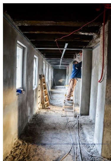
Works at the Borići site / IOM
